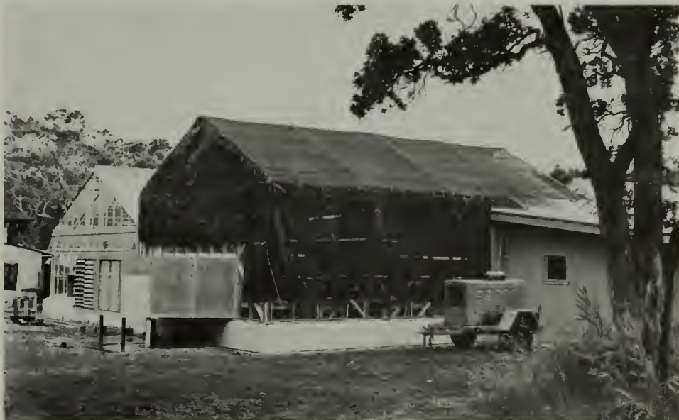
NPS quarantine facility at Hawaii Volcanoes National Park is designed as a greenhouse with natural sunlight and cooled by moving outside air through the secure area with large fans. The picture shadecloth is used in the summer to help control the inside temperature.
