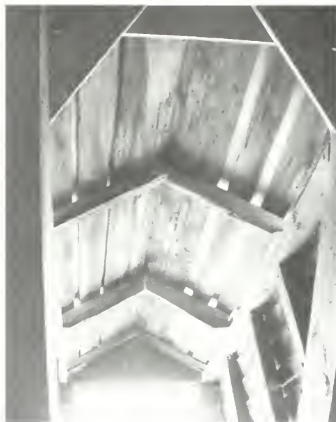
Figure 29 View of south dormer with original framing and decking intact. (NPS-SERO-CRS, 2001)
