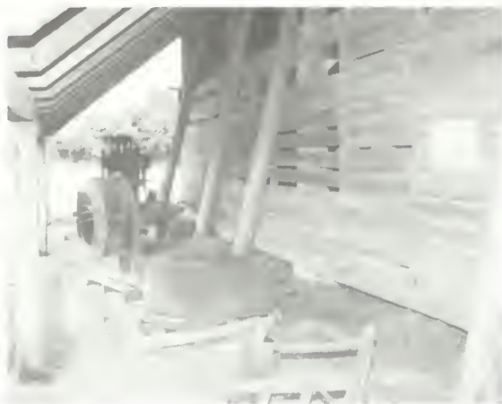
Figure 42 View west under south arcade, showing blowers and other equipment associated with c. 1900 system gin. (NPS-SERO-CRS, 2001)
