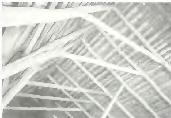
Figure 27 View of original pole-rafter roof in 1995. (NPS-SERO-Architecture, 1995)
