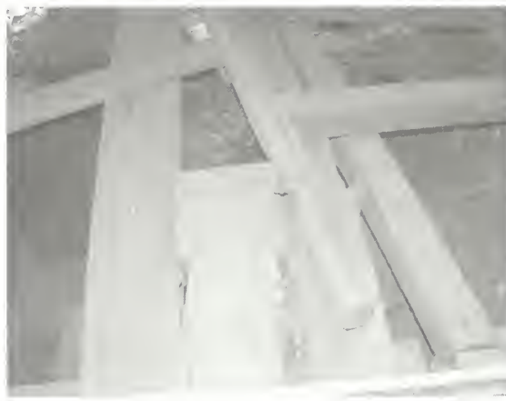
Figure 23 View of framing members in floor at east end of gin barn, with end of hewn beam visible at center, presumably from first cotton press. (NPS-SERO-CRS, 2001)
