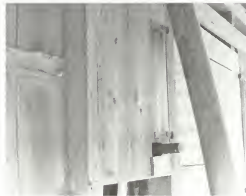
Figure 36 View of window H, which originally had sash but was closed when existing gin machinery was installed c. 1900. (NPS-SERO-CRS, 2001)
