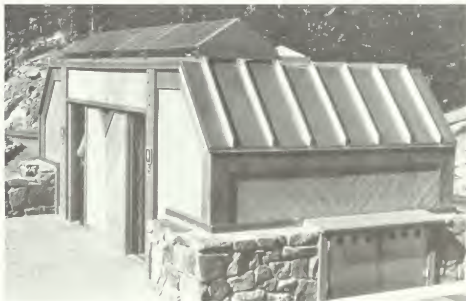
At Rocky Mountain NP, the photovoltaic unit to power the oil flush comfort station is designed into the structure.
