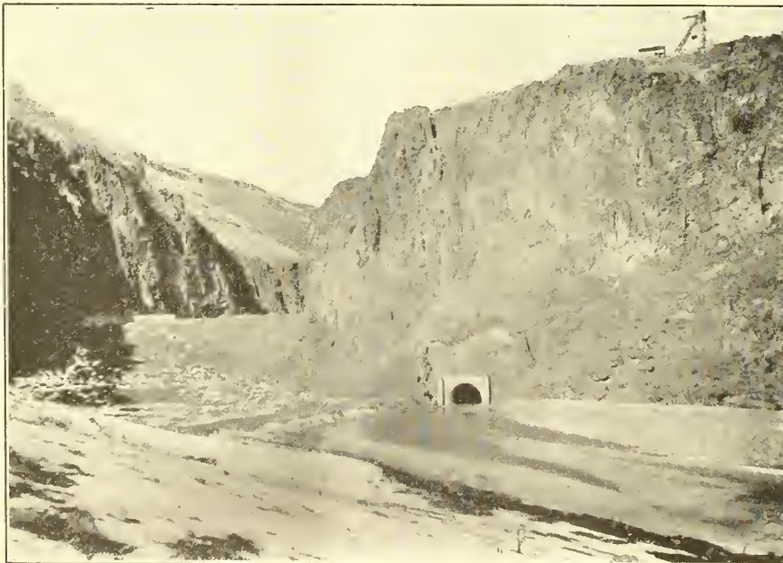
Upper cofferdam and diversion tunnel outlet from above Owyhee dam
