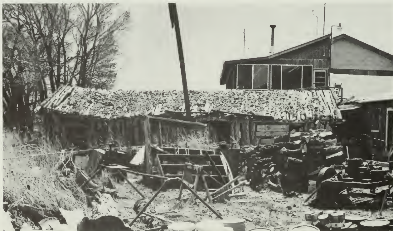
Fort Ruby, White Pine County, NV. This structure is the former Fort Ruby Headquarters and one of the only four extant pre-1870 log structures in Nevada. It is a rare example of palisade log construction. The structure has not been maintained and is in poor condition. New construction close to the historic log structures has altered their archeological and visual integrity. Photo: Holly Dunbar.
