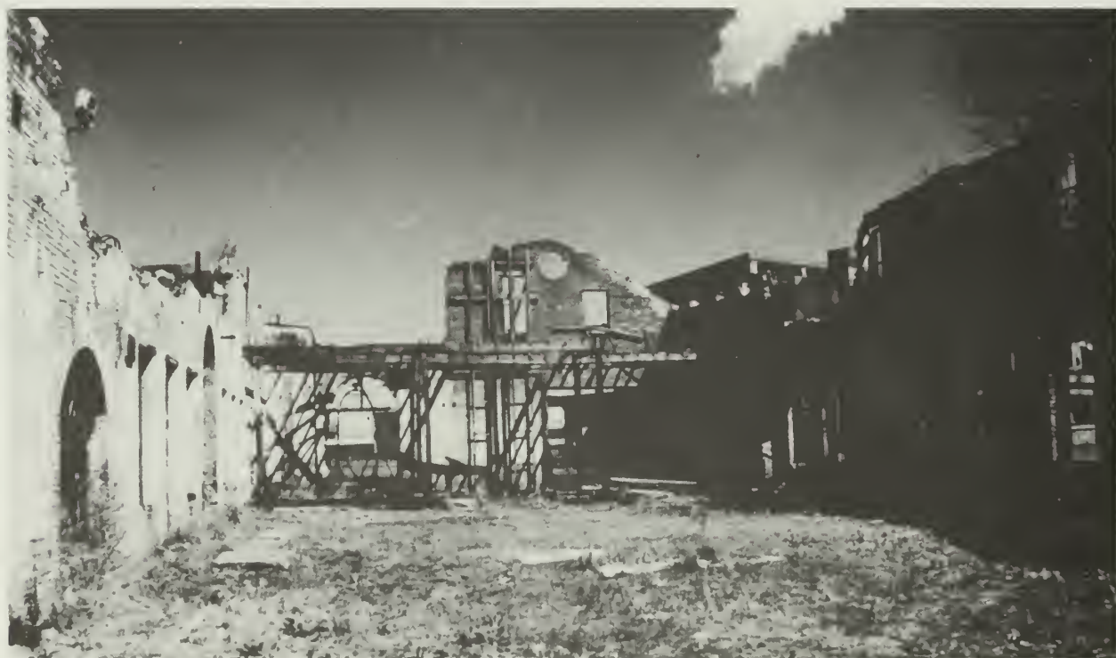
Central of Georgia Railroad Shops and Terminal, Savannah, GA. This Landmark is the oldest and best surviving example of a mid-19th century integrated railroad shops complex in the U.S. Although the head house and trainshed are in good condition, shop structures, as these illustrated, are vacant and severely deteriorated. Fires have gutted some shops, and in some cases destroyed large roof sections. Photo: Paul Hawke.
