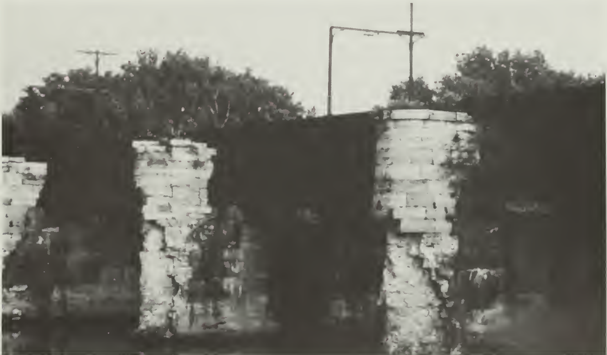
Illinois and Michigan Canal Locks and Towpath, Will County, IL. The canal linked Chicago to the Mississippi River, and completed a continuous waterway to New York City making Chicago a leading grain market and meat packing center. The canal encompasses locks and other engineering structures associated with the operation of the Canal. This illustration is of the Fox River aqueduct, the most seriously threatened structure. The structure is spalling, there are voids in the limestone, and it is in danger of collapsing. Photo: NPS Files.
