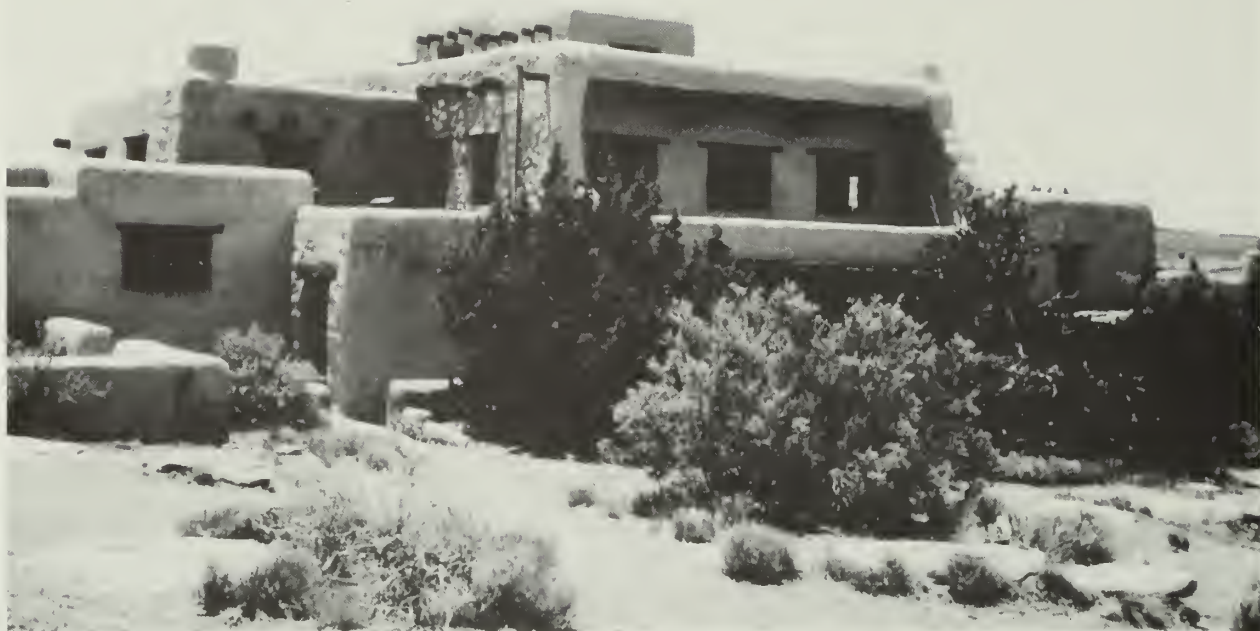
Painted Desert Inn, Petrified Forest National Park, AZ. This Landmark, built in 1937, is a Pueblo Revival style structure with highly notable interior features. Water penetration in the roof has caused structural damage and is beginning to damage significant interior murals. Photo: H. Ward Jandl.
