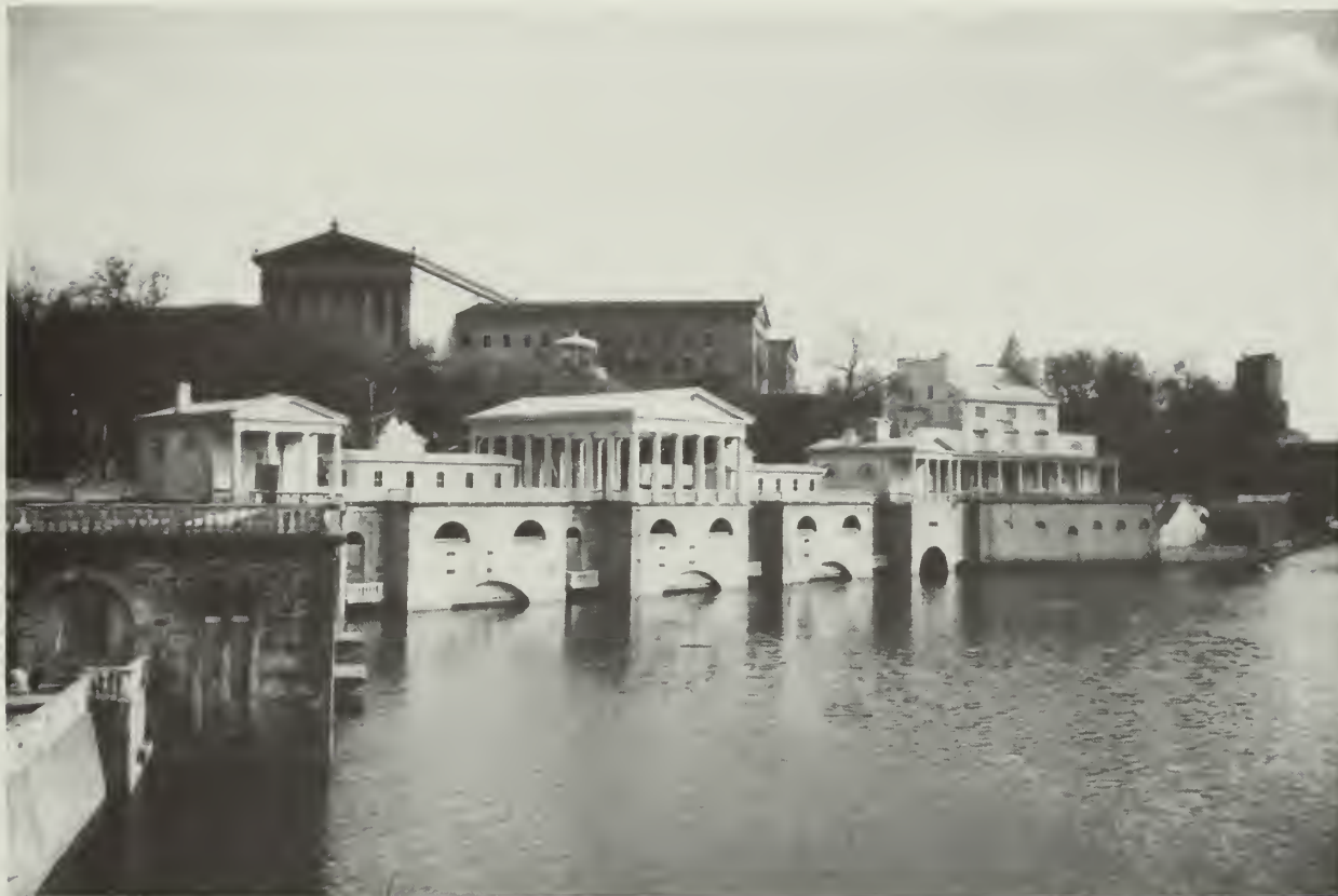
Fairmount Waterworks, Philadelphia, PA. These mid-19th century waterworks were the first municipal waterworks to use paddle wheels to pump water and the first to replace them with turbine engines. Above: Overall view of the waterworks. Most of the historic structures are being repaired or rehabilitated, however, the ca. 1860 mill house, in the left foreground, is sustaining extensive damage to its iron supports. Below left: Deteriorated ballustrade above the ca. 1860 mill house. Below right: Deteriorated columns at the Little Pavilion (not pictured in overall photo). Photos: Camille Martone.
