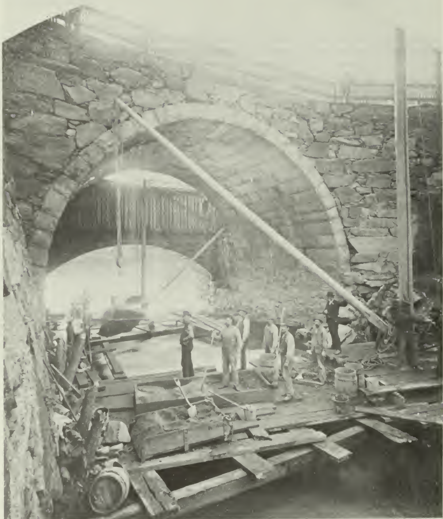
Repairing the abutments of the Prospect Street Bridge, Lawrence, Massachusetts, ca. 1895. Behind the bridge is the Spicket penstock. (MVTM Collections)
