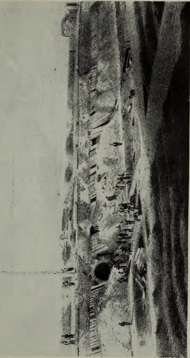
War-time sketch of the interior and rear wall of Fort Pulaski showing defense measures undertaken at the direction of Gen. Robert E. Lee on his last visit to the fort on November 11, 1861, to prepare the structure for the bombardment in April 1862; including the use of heavy timbers, or "blindages," earth embankments, and trenches in the parade to stop cannonballs
