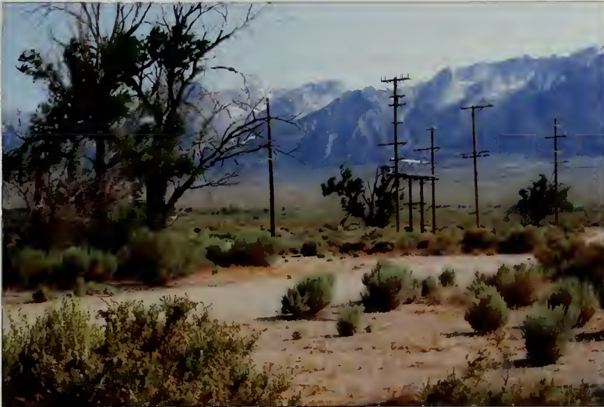
Figure 98. If feasible, non-historic utility lines at the military police compound should be relocated. (NPS, 2002)
