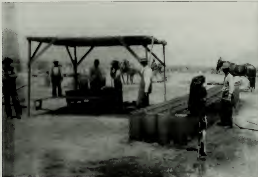
Figure 7. Concrete pipes were used to deliver water to orchards within the Owen's Valley Improvement Company irrigation colony at Manzanar. (Courtesy of the Eastern California Museum)
