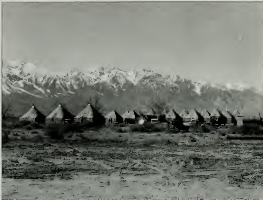
Figure 12. Before construction of the relocation center began in March 1942, military police camped in tents on the site. (Courtesy UCLA Special Collections)
