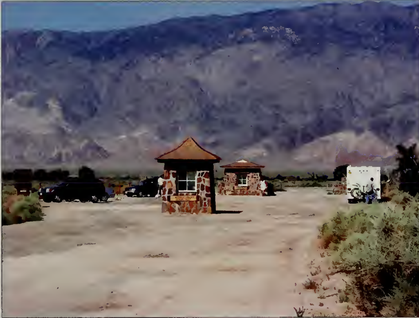
Figure 39. Internal Police Post (foreground) and Military Police Post at the entrance after restoration work. (NPS 2001)
