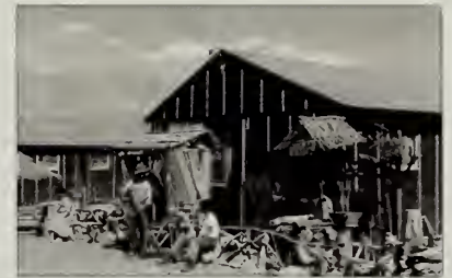
Figure 28. Using limbs and other found objects, a variety of structures such as awnings were built to shade barrack apartments from the hot summer sun. The Takemura family residence, shown here, was one of the more elaborately embellished barrack buildings at Manzanar. (Courtesy of the National Archives and Records Administration)
