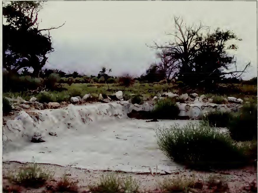
Figure 123. Stabilize and interpret unique historic features like the wading pool in the demonstration block. (NPS, 2002)
