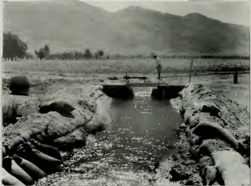
Figure 87. An extensive system of open ditches supplemented with pipes carried water to irrigate fields. (Courtesy of the National Archives and Records Administration)
