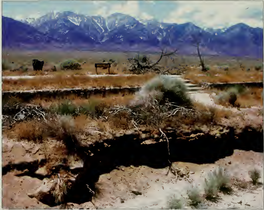
Figure 113. Stabilize eroding soil that threatens site features. (NPS, 2002)
