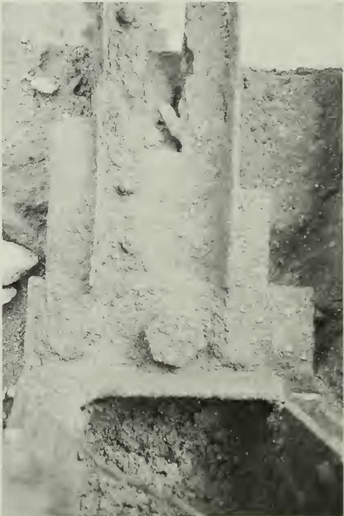
Figures 2 and 3. The extent of damage can be seen in the bent vertical post member (below, left) and the heavily corroded end post (right). Similar problems existed throughout the structure. Photo: Beta Engineering.
