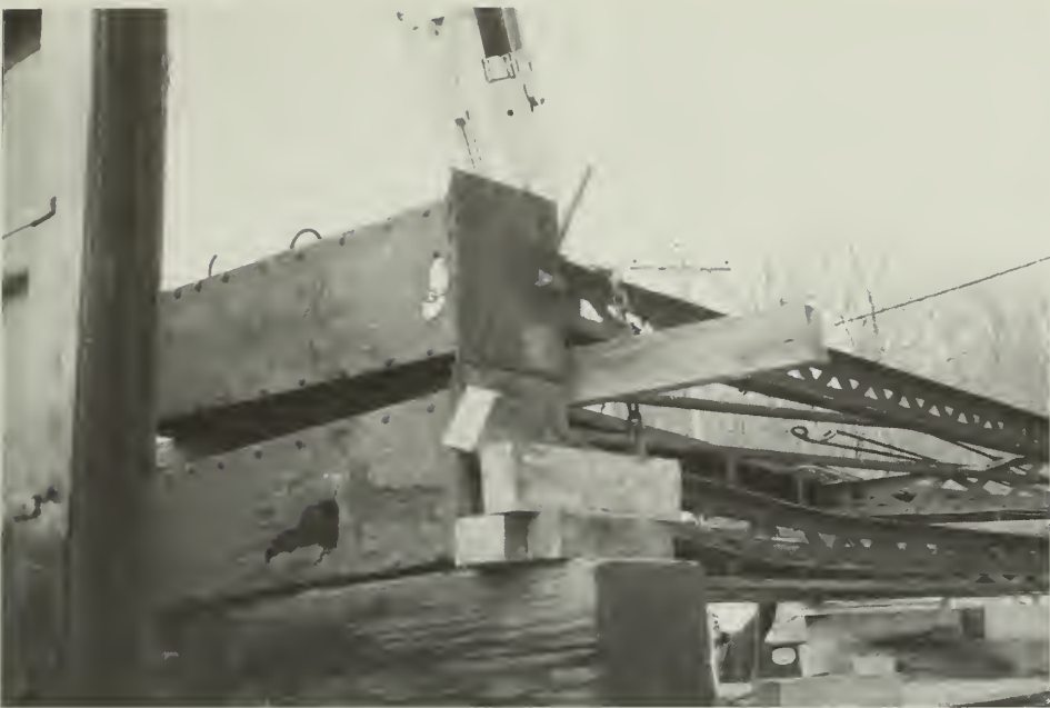
Figure 6. Although plans specified that the trusses be placed in an upright position, they were placed on the truck on their sides (left). The lower truss was damaged during the loading operation. Photo: Beta Engineering.
