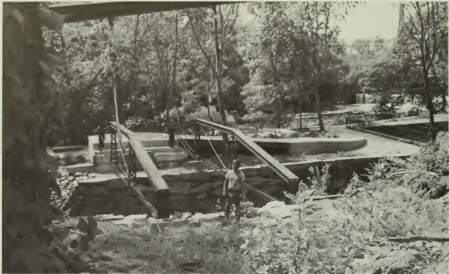
Figure 9. The trusses were lifted by crane and set into position on the new site. Photo: Beta Engineering.
