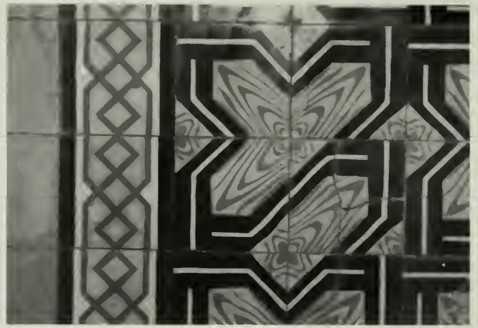
Figure 16. Historic cement floor tiles in a house at 103 Calle San Jose, Old San Juan, Puerto Rico, feature a design intended to resemble wood parquet. (Note the mismatched repair.) Photo: Jack E. Boucher, HABS Collection.
