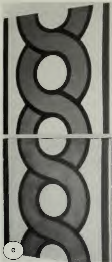
(e) The top tile is a new reproduction of the historic tile below. (f) This design is identified as No. 84 in Miller & Coates' Minton Tile Catalogue (detail Figure 2). (g) What might appear to be an inappropriate repair with non-matching modern tile in the center of the star is, in reality, a neatly executed patch to serve as temporary in-fill for the reproductions that have been ordered. (h) Shown below is a restored section of the Capitol floor. Photos: (e,g,h) Wayne Firth, Office of the Architect of the Capitol; (f) David W. Look, AIA.
