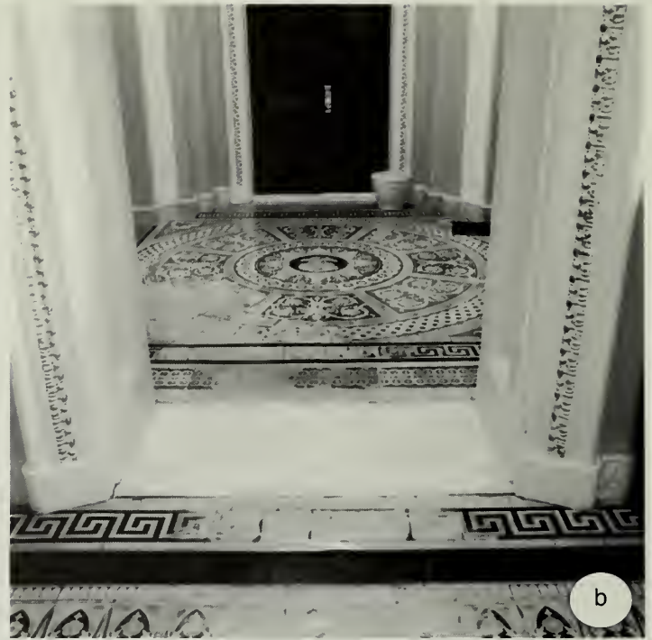
(a-b) Above: By the mid-1970s, many of the patterns in the encaustic tile floors had become faint, and some had completely worn off in the most heavily trafficked areas. (c) Below left: Damaged areas of the floor had been patched with salvaged pieces of tile that fit, but did not match. Photos: Wayne Firth, Office of the Architect of the Capitol.
