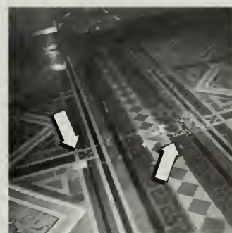
Figure 21. These cracked geometric tiles may have been damaged by the repeated passage of heavy equipment over the floor. Photo: Anne Grimmer.
