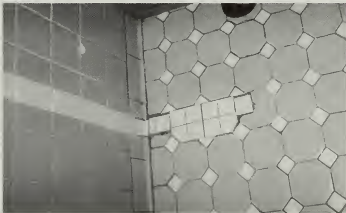
Figure 23. These non-matching tiles are inappropriate replacements for original tiles that were damaged during bathroom remodeling. Photo: Anne Grimmer.
