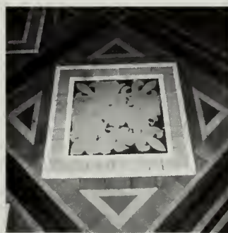
Figure 20. The surfaces of these late-19th century encaustic tiles have become worn and much of the pattern has been lost after more than 100 years of use. Photo: Anne Grimmer.
