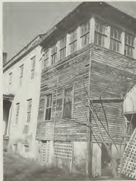
Pemberton's Headquarters, Vicksburg, MS. This house was the headquarters of Confederate Commander Lieutenant General John C. Pemberton during most of the siege of Vicksburg, and the place where the decision to surrender the city was made on July 4, 1863. The building is severely deteriorated and has suffered considerable water damage. Above left: West facade with missing bricks and mortar. Above right: Circular stair with rotting woodwork. Below left: Damaged plaster walls and ceilings. Below right: Southwest corner with rotting siding and damaged roof. Photos: Paul Hawke.
