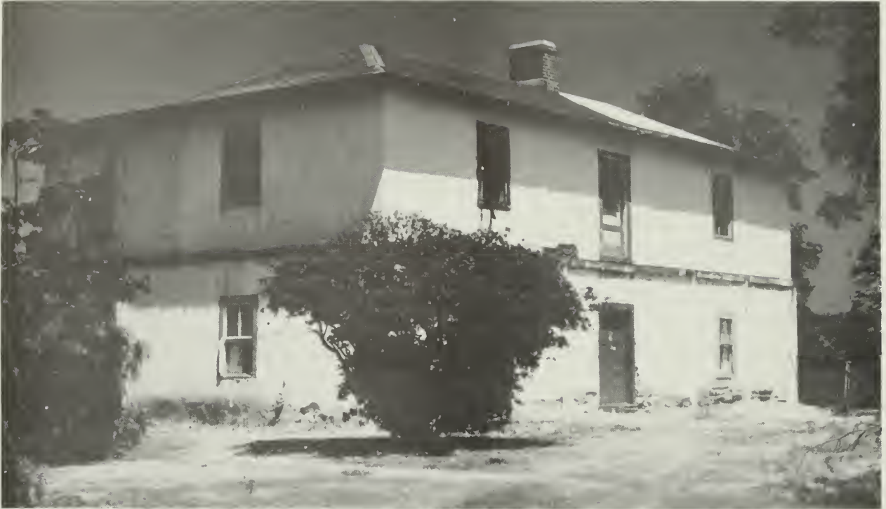
Las Flores Adobe, Camp Pendleton, CA. This ranch house is a prime example of a two-story 19th century Monterey Colonial style residence, a popular building type unique to California during the mid-19th century. The house is in a very deteriorated state. Adobe is crumbling, floors are damaged, and a veranda was removed due to termite damage. Photo: Ann Huston.
