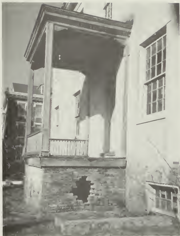
Pemberton's Headquarters, Vicksburg, MS. This house was the headquarters of Confederate Commander Lieutenant General John C. Pemberton during most of the siege of Vicksburg, and the place where the decision to surrender the city was made on July 4, 1863. The building is severely deteriorated and has suffered considerable water damage. Above left: West facade with missing bricks and mortar. Above right: Circular stair with rotting woodwork. Below left: Damaged plaster walls and ceilings. Below right: Southwest corner with rotting siding and damaged roof. Photos: Paul Hawke.
