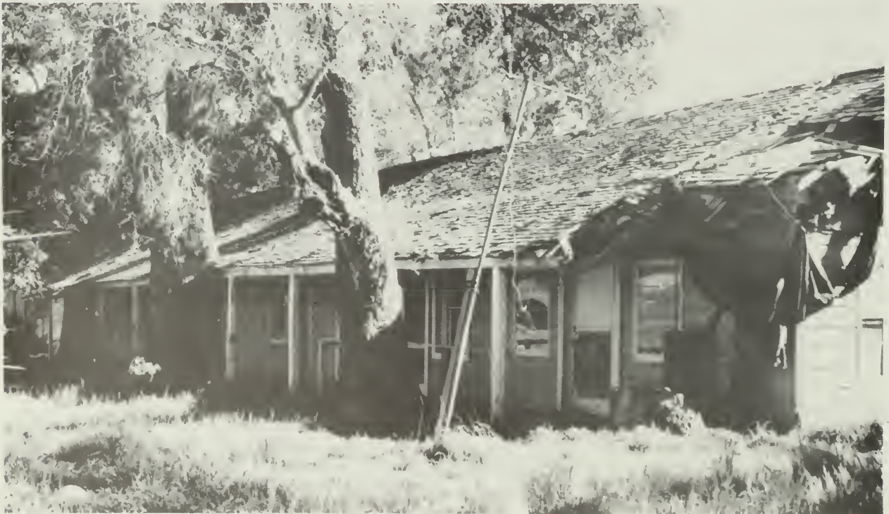
Oak Grove Butterfield Stage Station, Aguanga, CA. This stage station is one of the only remaining stations on the Butterfield Overland Mail Route which operated between San Francisco and two eastern terminals from 1858 to 1861. The building has been vacant and without maintenance for several years. The roof has partially collapsed and adobe is crumbling. Photo: Ann Huston.
