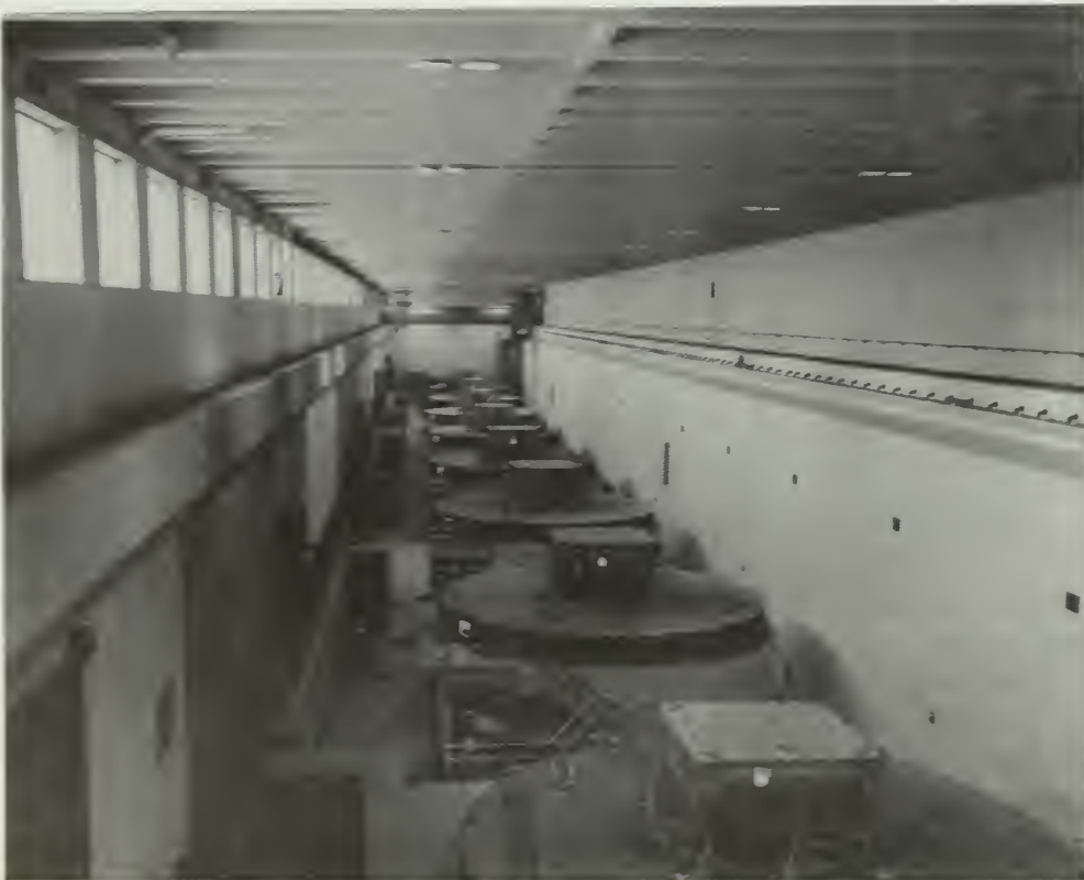
Generators in a dam powerhouse
