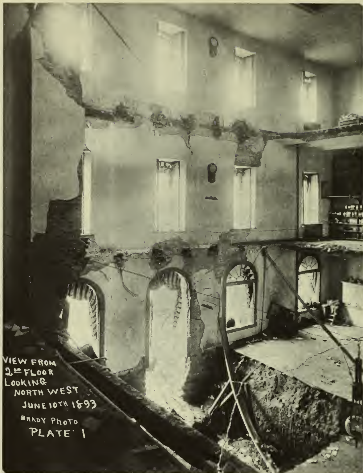
FIGURE 52. Interior of Ford's Theatre building after partial collapse in 1893, showing inside view of original casement windows and unexcavated basement.
