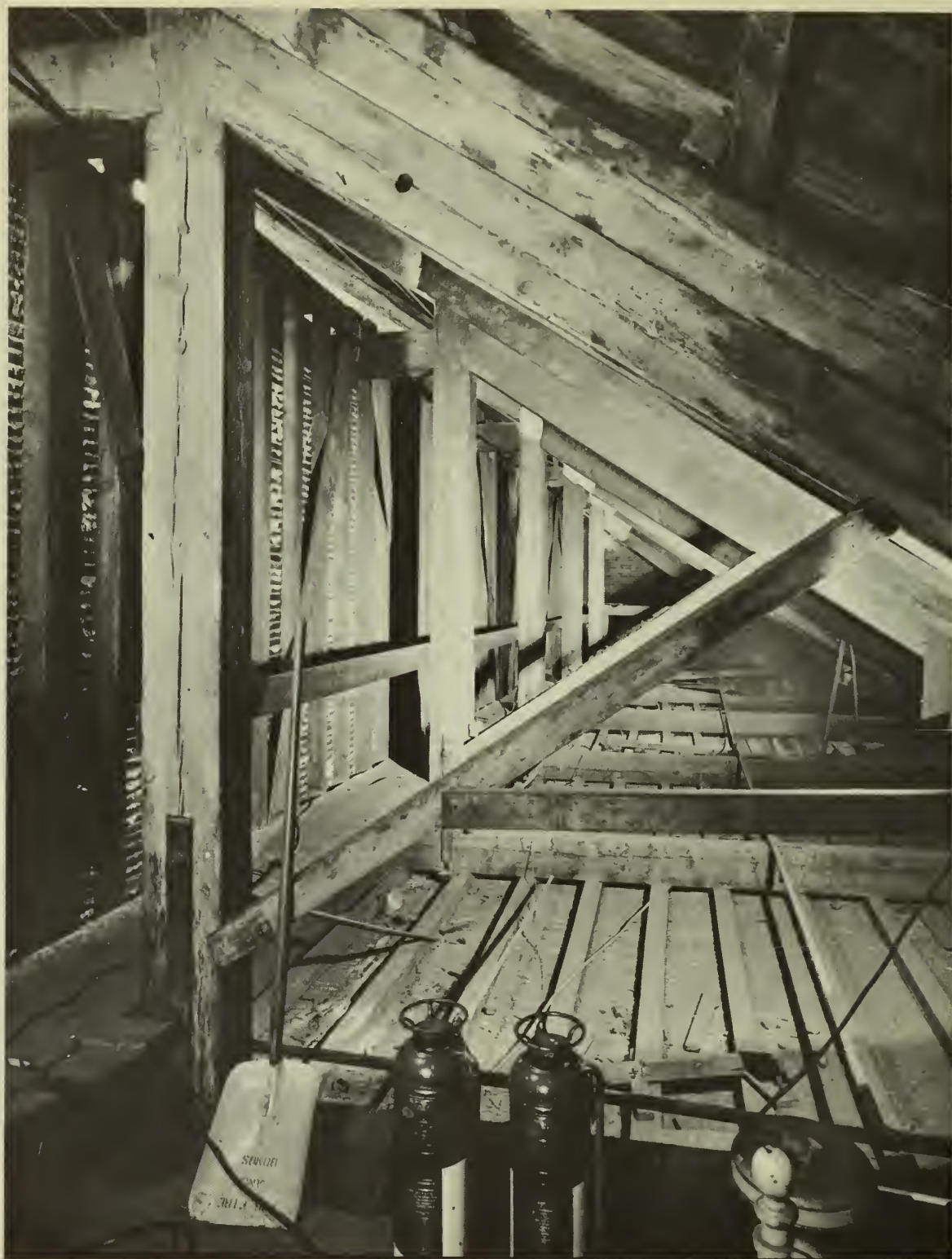
FIGURE 15. Original wooden roof trusses still in use, Ford's Theatre, August 1963.
