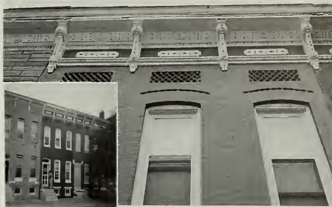
Figure 18. As part of an urban housing grant program, the exterior of this row house was successfully made lead-safe and met the Secretary of the Interior's Standards for Rehabilitation. The exterior was washed, then repainted with exterior grade alkyd paint. The decorative roof brackets and cornice were repainted; not removed or covered as is often recommended in typical abatement guidelines. The previously altered, deteriorated window sash were replaced with new sash and jamb liners set within the historic frames. Photos: Deborah Birch.
